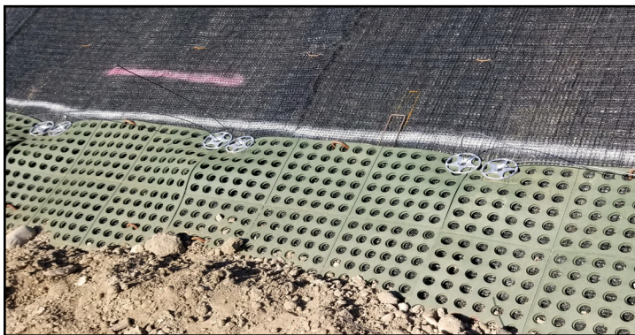
ShoreMax mat installed at toe of slope with ground anchors (left), Permanent P550 TRM placed on slope surface and anchored with PDAs for upper slope stabilization (right).
