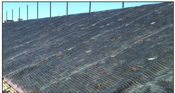
ShoreMax mat installed at toe of slope with ground anchors (left), Permanent P550 TRM placed on slope surface and anchored with PDAs for upper slope stabilization (right).
