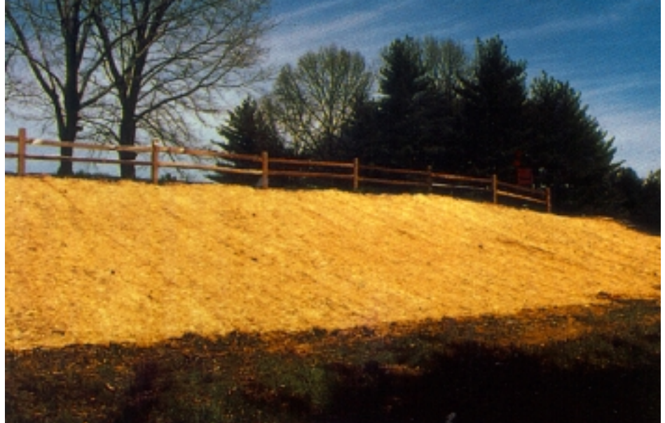
Erosion-control fabrics, when properly used, can offer superior erosion control on slopes subjected to heavy rainfall. File photo.
