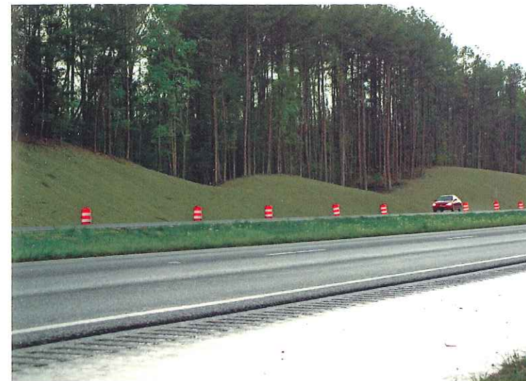
Crews applied HydraCX 2 mixed with a standard summer seed mix over land comprised of sand, rock, and clay and reaching slopes of 3:1 and greater.
