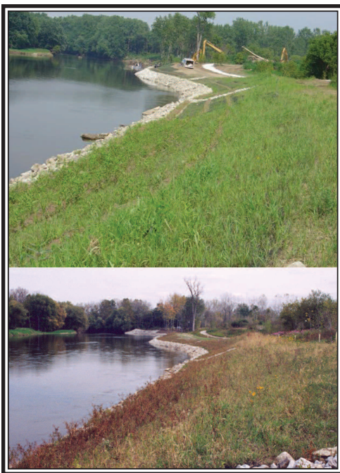
Vegetation is nearly fully established on the river banks in only three months (top), and a mature vegetation stand (bottom) offers a diverse array of native species for wildlife habitats. The soft armored P550 C-TRM saved the city $800,000 compared to 30" rock rip rap.
