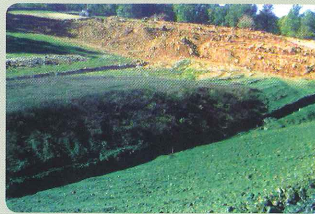
When straw blankets blew away in windy conditions, TDOT introduced a hydraulically applied blend.
