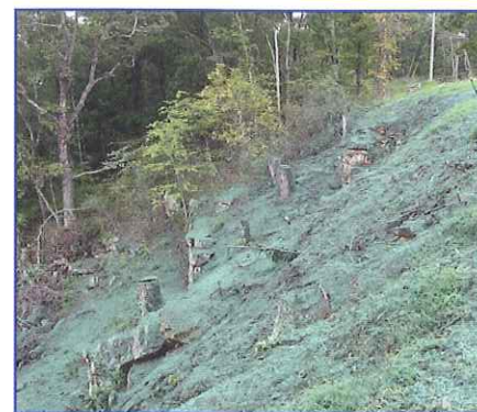
Applied using a one-step method, the mulch was applied at 3,000 lbs. per acre.
