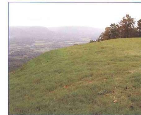
Complete grass growth was established able to withstand the erosive forces from weather and aggressive activity by paragliders.
