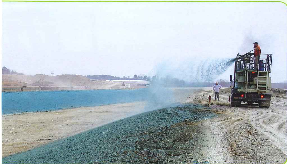
The project's erosion control specialist discovered improved tank load efficiency using the third hydraulic mulch solution.
