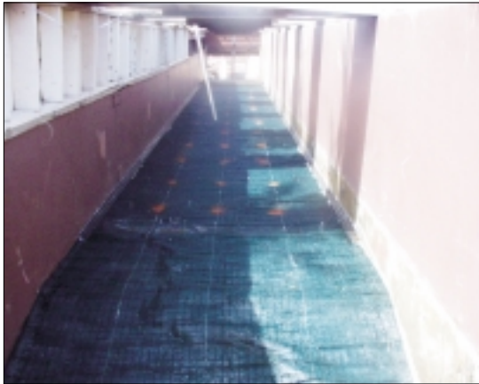
The surface applied Vmax 3 mats after installation in test flumes.
