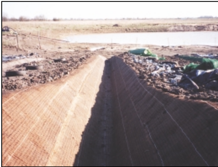
Figure 4. The C350 just after surface application in the test channel.
