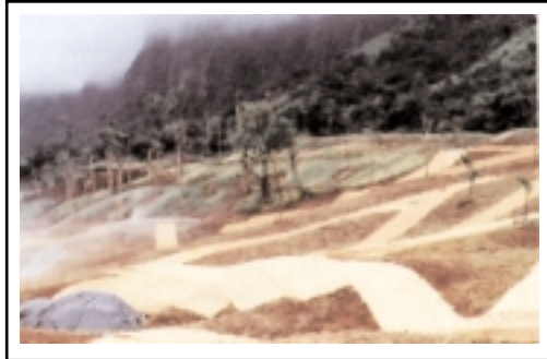
A maze of North American Green erosion control blankets trace runoff at Minami. 40 GPM sprinklers and heavy rains necessitated the use of erosion blankets to prevent rill and gully formation.
