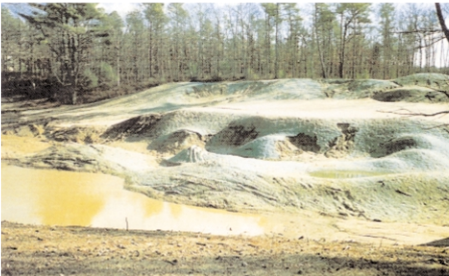
Failure to use the most effective erosion-control method can have disastrous results.
