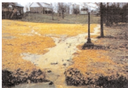
Loose mulches without sufficient anchoring will not be as effective at preventing erosion in areas where water flow concentrates, compared with hillside areas of less concentrated water flow
